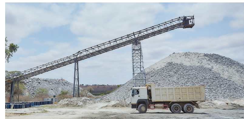
Above: Commissioning of Eureka Gold Mine.
